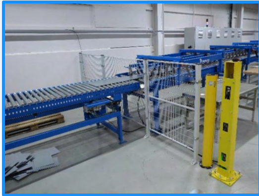
Detailed sheets can continue on to roll forming or be removed for further processing.
